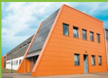
Solar power plant, Johanna Solar
